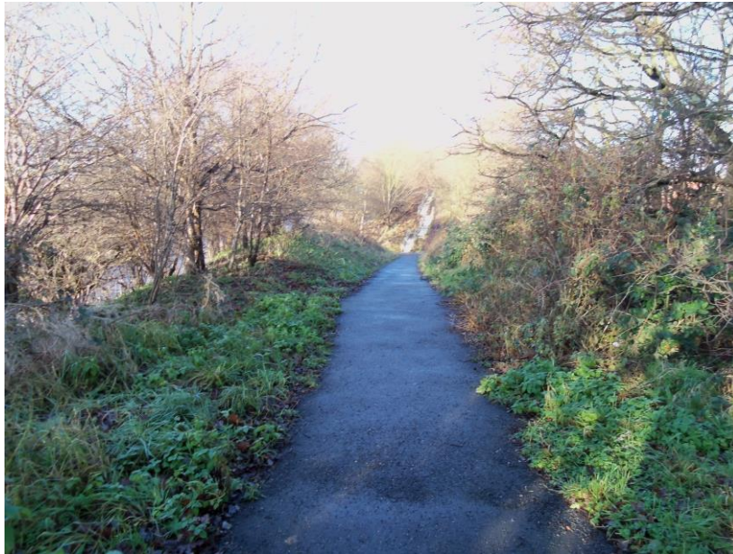
Figure 3: part of the surface improvements along the disused rail corridor
