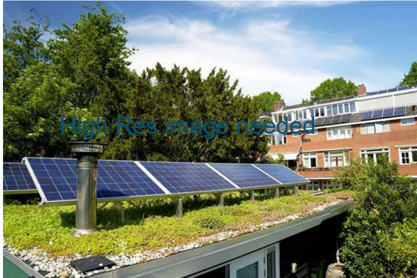
Figure 5: Example of a biosolar roof
